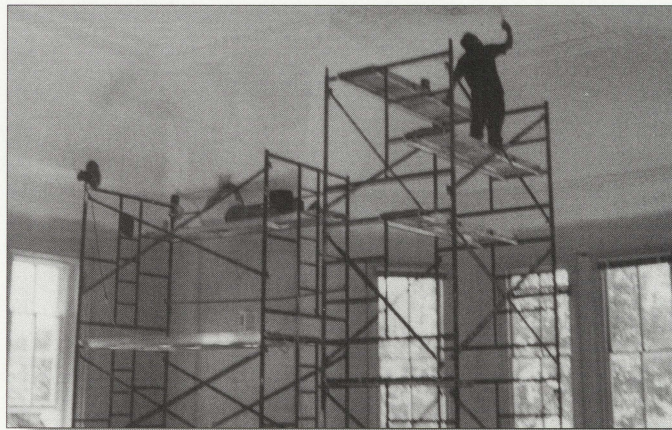
A worker puts finishing touches on the newly refurbished pressed-tin, domed ceiling in an office adjacent to the enclosed walkway to the chapel in Chapel Hall.
